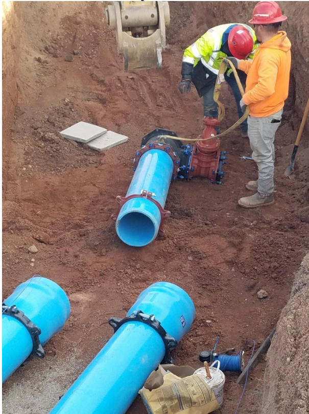
Installation of T Assembly:
