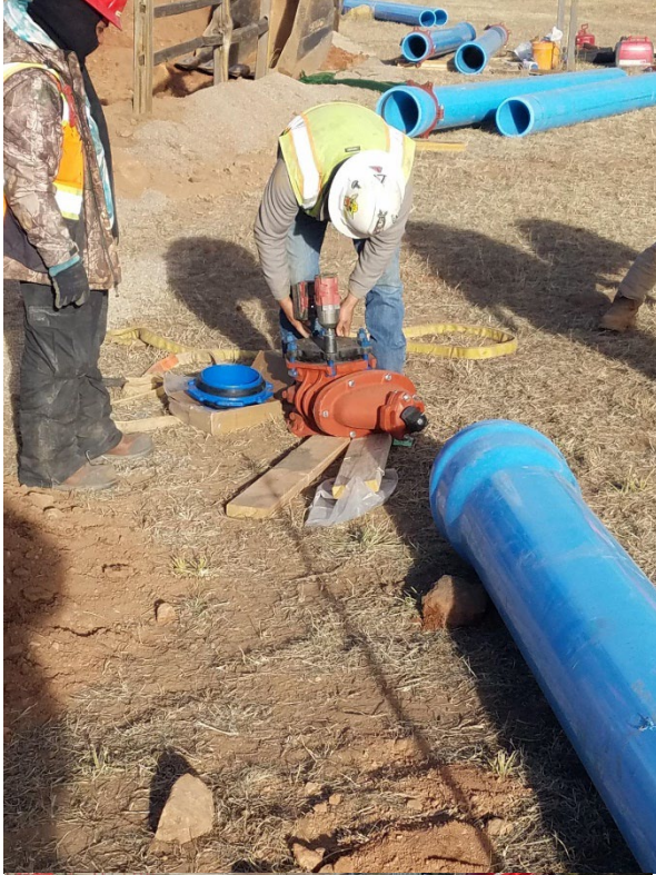
Assembling the 12"x8" T, Foster adapter, 8" Gate Valve and 12" DR-14 C100 PVC Pipe:
