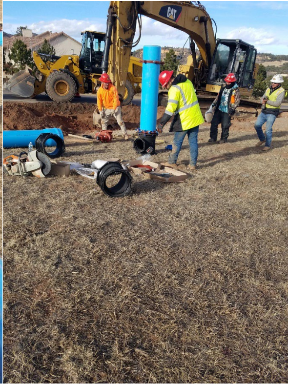
Assembling the 12"x8" T, Foster adapter, 8" Gate Valve and 12" DR-14 C100 PVC Pipe:
